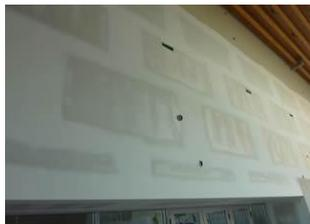
Ever hear this one? This paint inspector walks onto a jobsite and sees a drywall surface that's just been meticulously painted with an intermediate coat of premium high performance interior latex...and his stomach turns: the wall looks awful, with the joints clearly visible at both the bevel joint seams and butt joints. The architect and owner are upset and the painting contractor is pointing at the drywall contractor. The drywall contractor, however, insists the work was done to spec.
